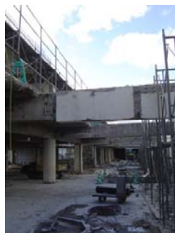
Demolition of the part of the Path of Light
