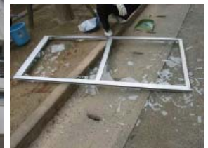
Fallen and broken window frame
