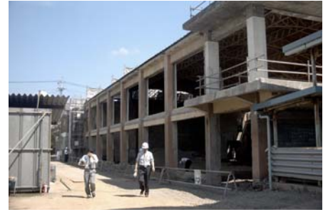
Figure 4: Scenes during refurbishment
