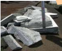
Fallen mortar due to deterioration
