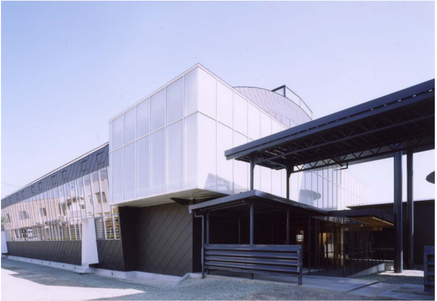
Indoor gymnasium after refurbishment
