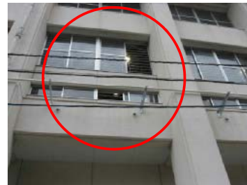
The window's original position
