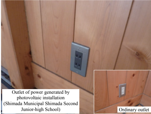
Installing outlet for power generated by photovoltaic installation
