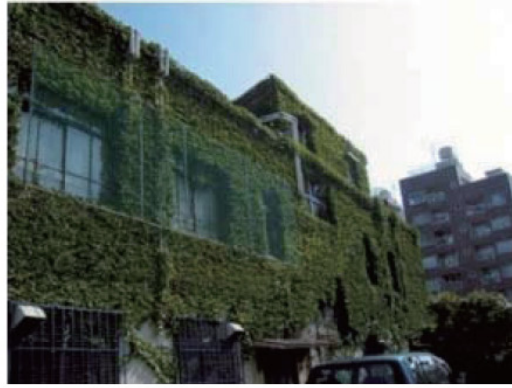
Wall vegetation (Climbing type) Source: Wall Greening Guideline, Tokyo Metropolitan Government
