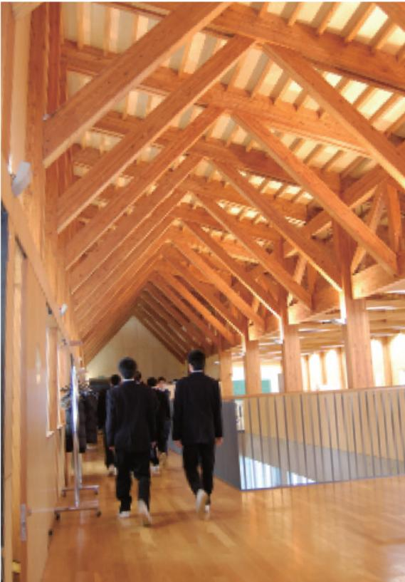
1 East side of the south building 2<sup>nd</sup> floor. Students can learn in a space full of the warmth of wood under a continuing frame made of glued laminated timber with large dimensions.
