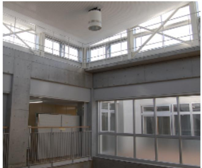
7 Balance windows installed for natural ventilation in the upper part of the Media Court relieve the heat in summer to maintain a comfortable room temperature.
