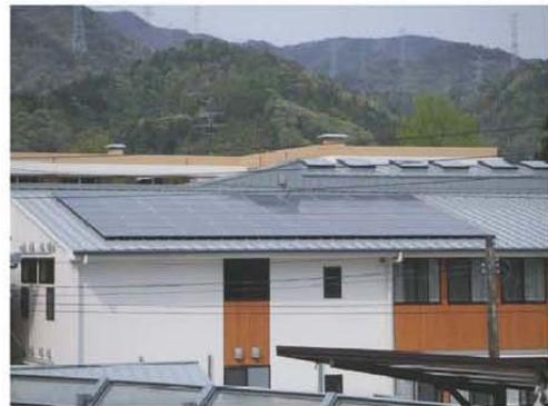
Solar cell modules installed almost flat on a pitched roof
