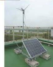
Wind power/ photovoltaic hybrid power generation facilities: Wind power is used on cloudy/rainy days.
