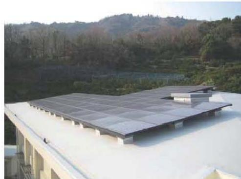
Mounting frames were not used, even though the roof is almost flat
