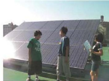
Solar cell module facing south, fixed at a tilt angle of 30°
