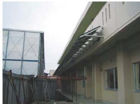
Solar cell modules serving as eaves were installed on an existing school building.
